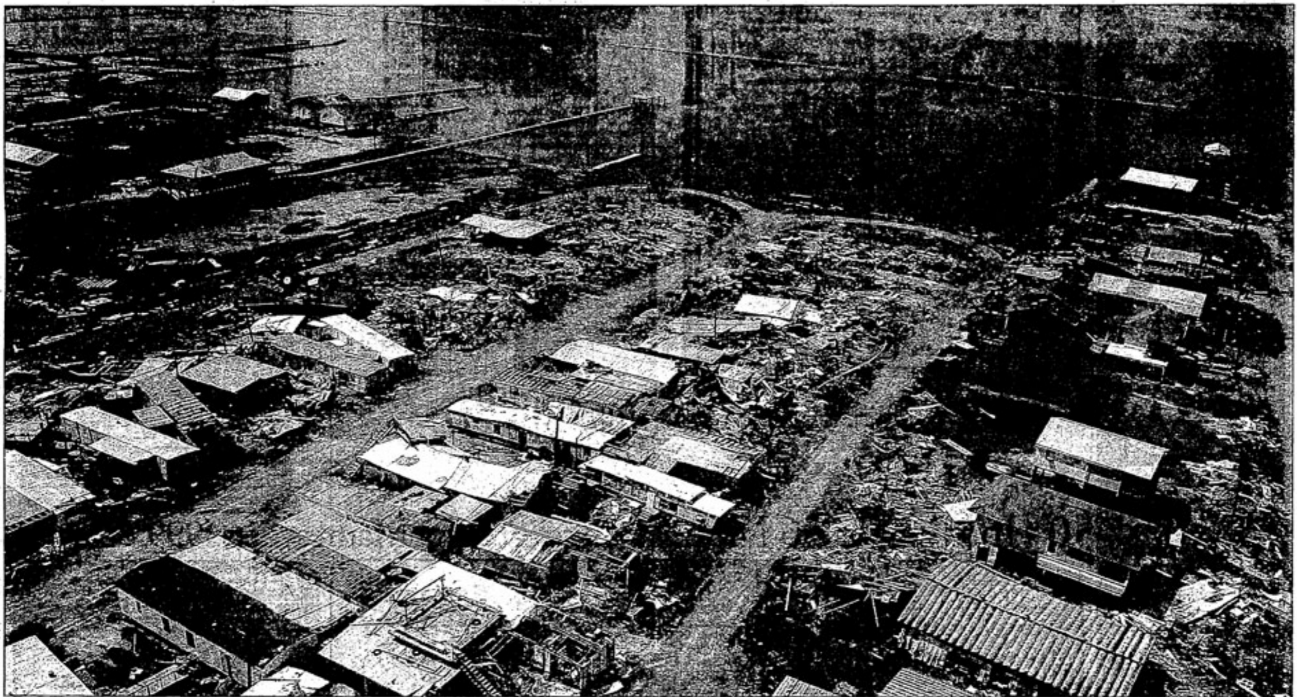
Hurricane Katrina caused catastrophic damage to 70 percent of Grand Isle's structures, Fire Chief Aubrey "T-Black" Chaisson said Friday. A small group of full-time residents have been working during the day trying to clean up and repair the damage.
